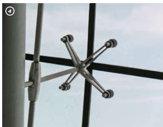
4: Quattro node 350 x 350 mm for glass panels 2500 x 2500 mm. Glass Cube Banco Santander, Madrid (see cover & page 6, 7)
