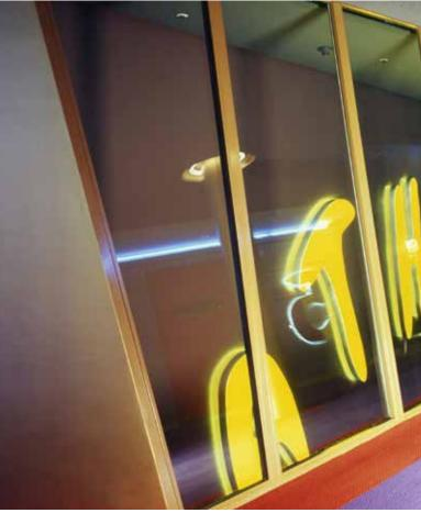
An important feature of FIRESWISS FOAM, the El classified fire protection glass manufactured by Glas Trösch, is the protection it offers against dangerous radiated heat. Thanks to a so-called protective heat shield, radiant heat is reduced allowing people and rescue services a safe passage along emergency and escape routes. Depending on the requirement and glass type used, fire resistance of up to 120 minutes can be achieved.
